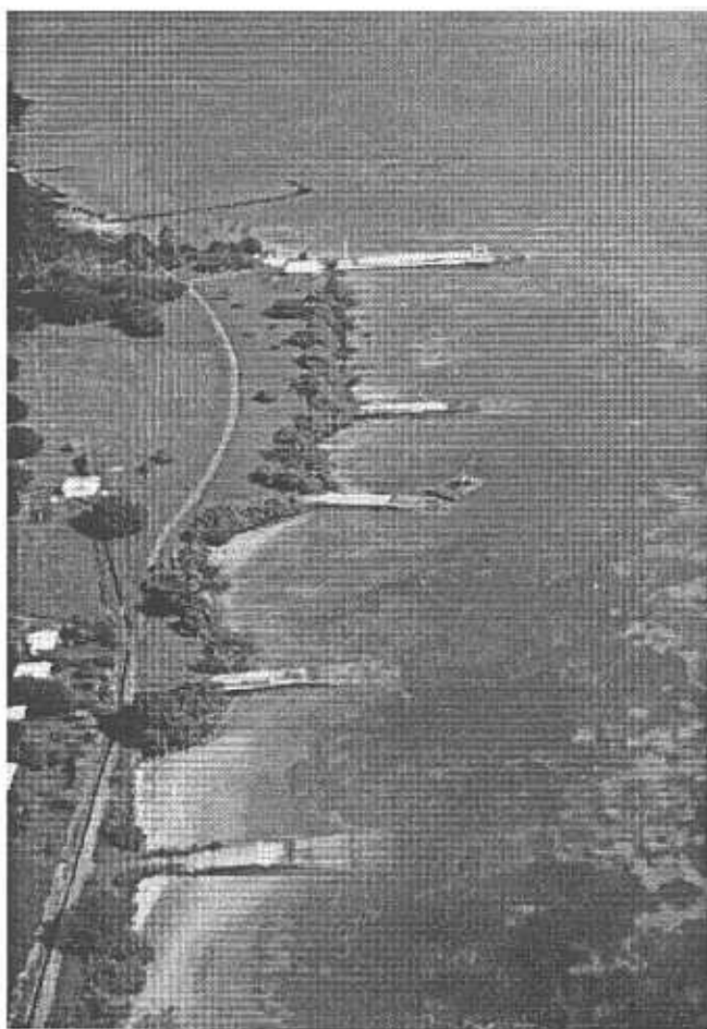
Figure AI/1. Top: a) Shoreline near Lalovi, Mulifanua showing eroded coconut palms on shore, basalt boulders (foreground) used in revetment to protect coast road, and reclaimed land with fale in centre. View to south. Bottom: b) Oblique aerial photograph near Toloa showing groins and dragline. Note the general lack of sediment on the beach; the groin at the bottom has trapped some carbonate sand on its eastern side indicating transport to the west. The darker areas on the reef flat is covered by marine flora. View to west.
