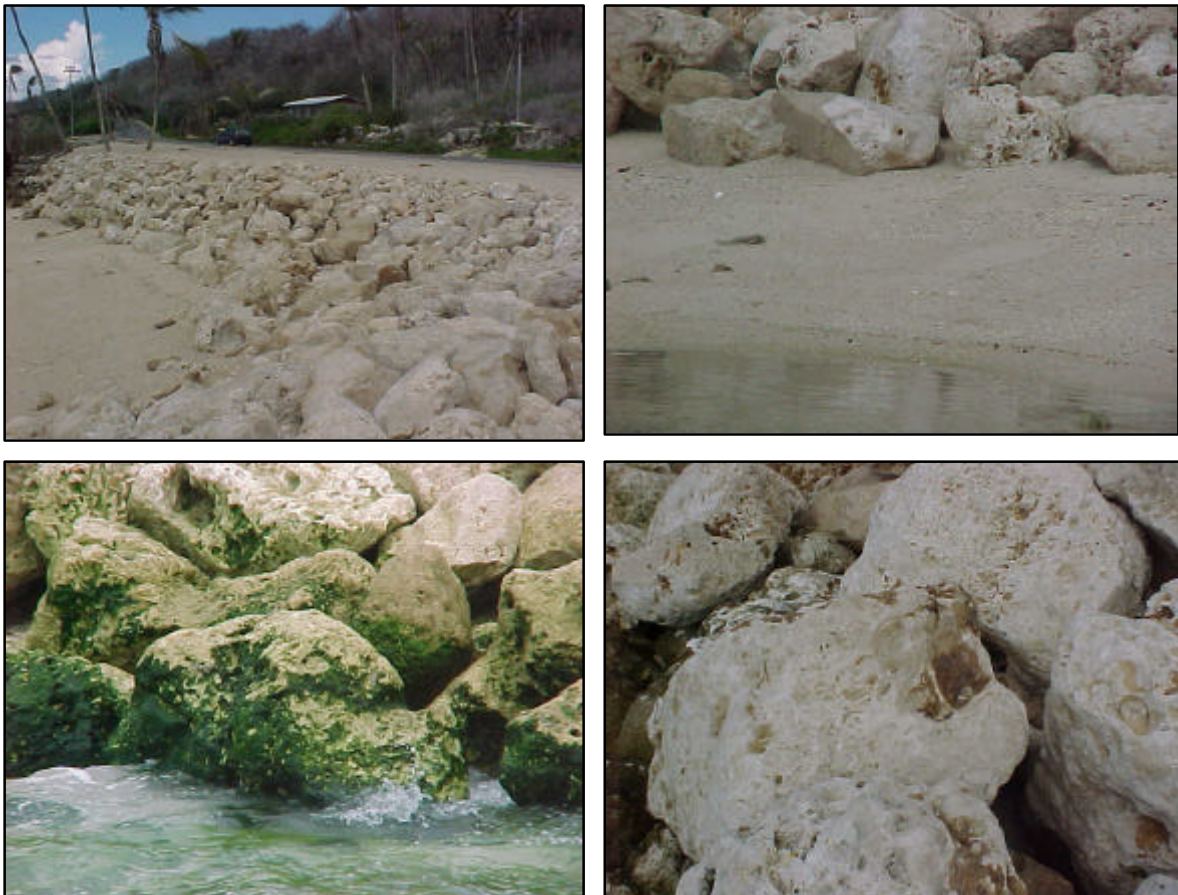
Figure 22. Rip-rap characteristics at the harbour site. Top left – a single-layered rip-rap, protecting an eroded segment of road, on the Southern side of the harbour; top right – rip-rap at the toe of the groin; lower left – algae-covered rip-rap at the toe of the groin, alongside the mooring basin; and lower right – note rip-rap boulder shape, angularity and pits.
