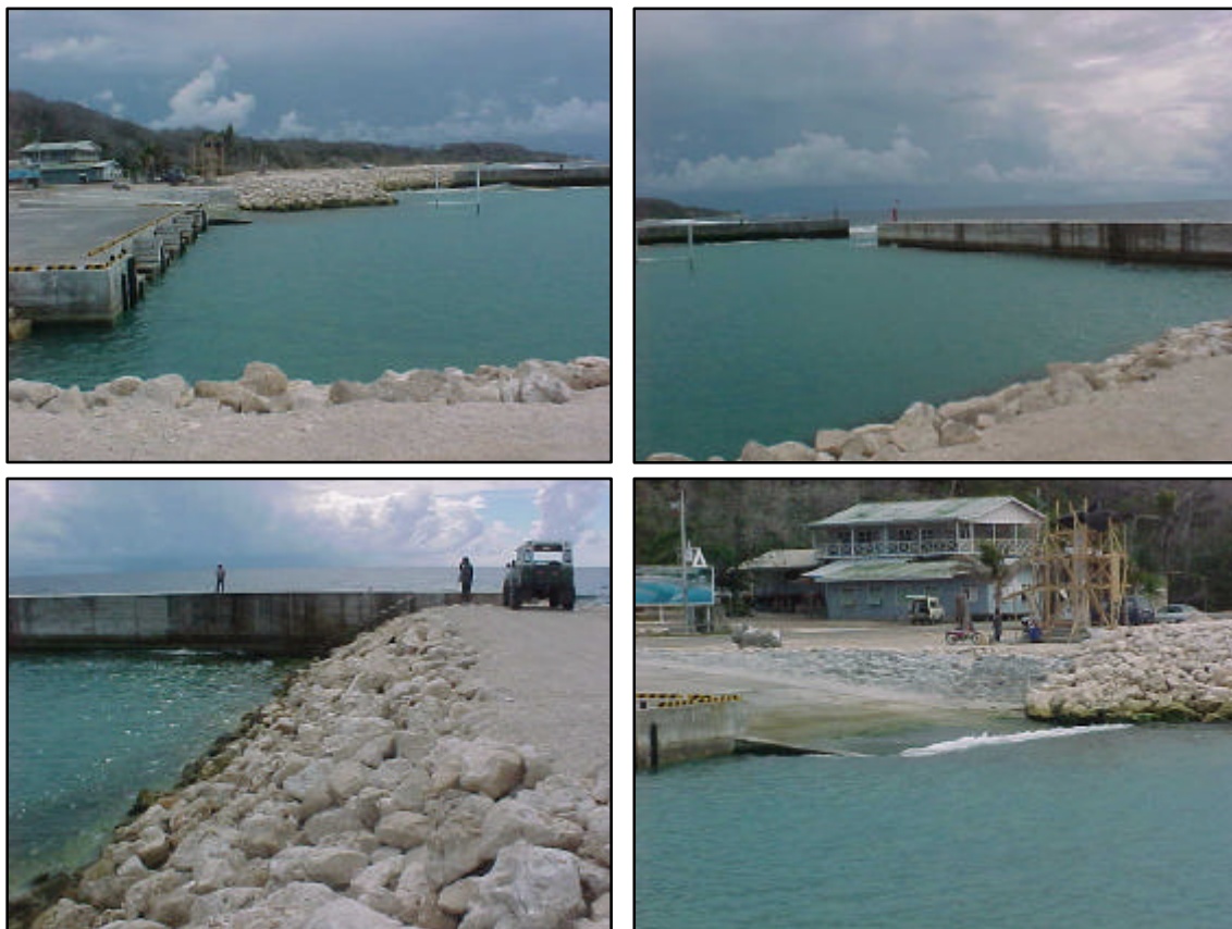
Figure 20. Characteristics of the new harbour facility. Top left – mooring basin/wharf, with quay wall and apron on left of the photo; top right –sub-breakwater and main concrete breakwaters (left and right respectively); lower left – rubble groin, with rip-rap and main concrete breakwater; and lower right – concrete boat ramp, with rip-rap pitched spending slope on the rear right.
