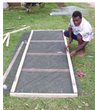
2. Stretching the chicken wire on the frame
