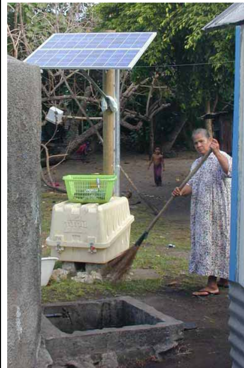
Figure 4.5 - PREFACE SHS installation
