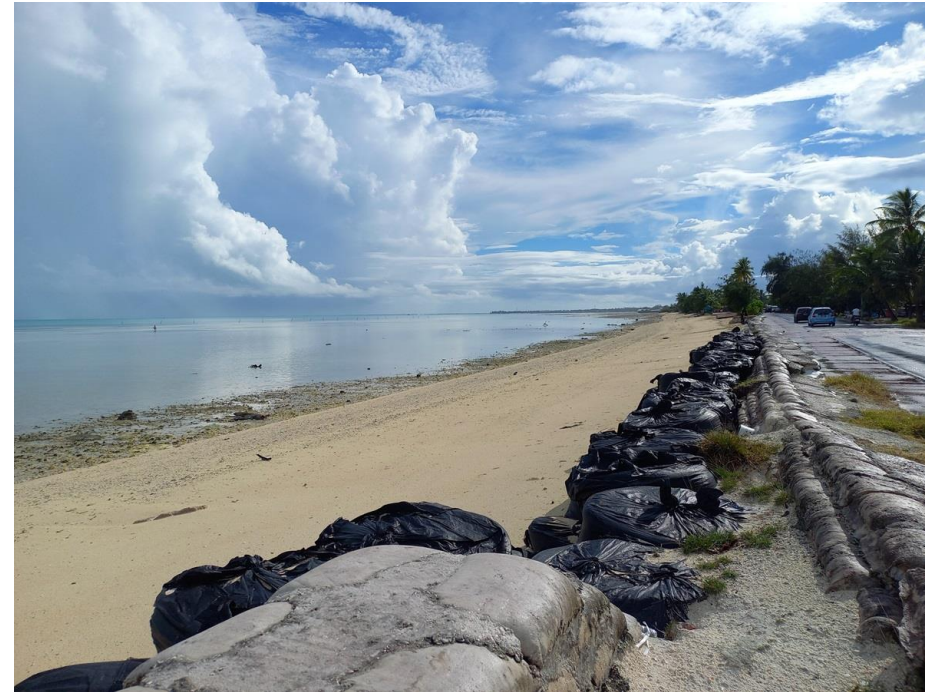
Sea-level rise impacting Kiribati ©Sangeeta Mangubhai
